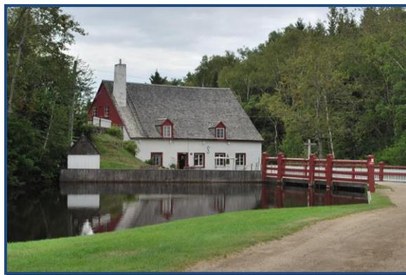
Last July, we began the restoration project of the Les Éboulements Mill. The work consisted of north side roof repairs (cedar shingles), front attic windows, front wall and the wall on the south side.
