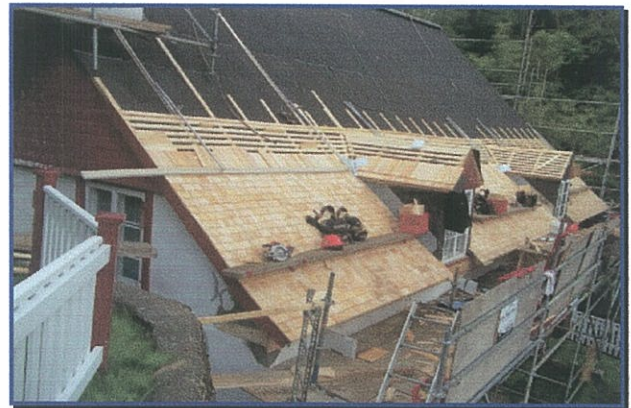
Using battens to provide ventilation under shingles
